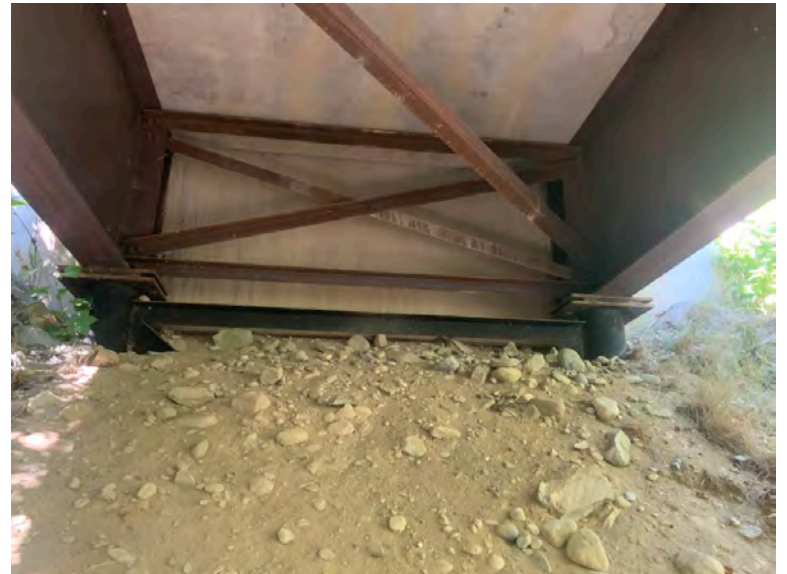
Left Bank Abutment when facing downstream
