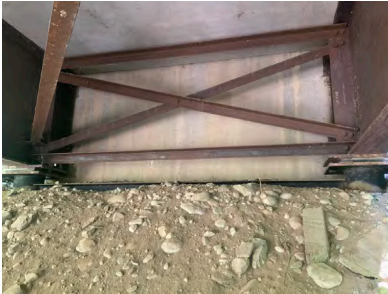
Right Bank Abutment when facing downstream
