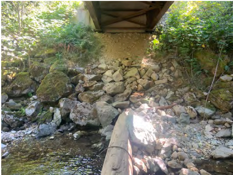
Right Bank Abutment when facing downstream
