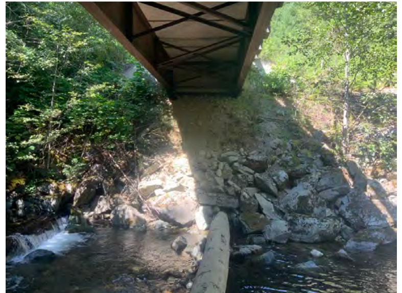
Left Bank Abutment when facing downstream
