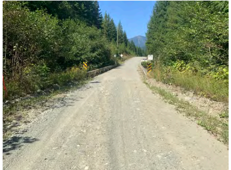
Right Bank Abutment when facing downstream
